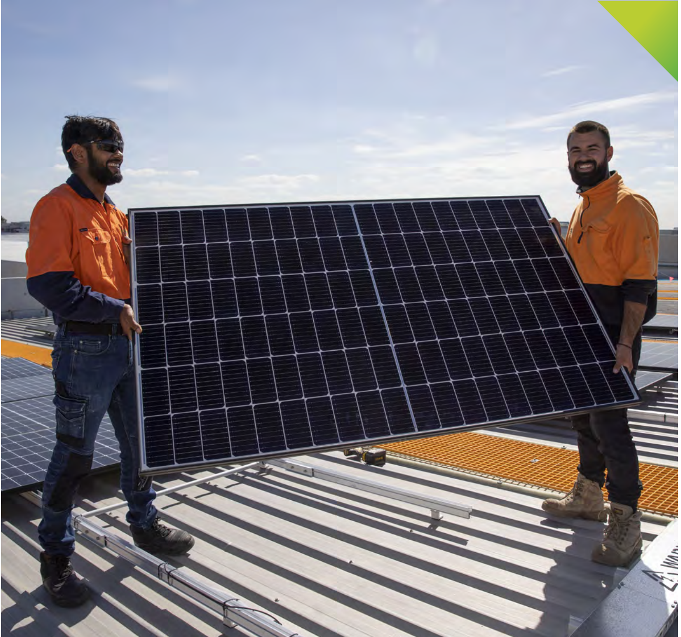
Credit: Solar Victoria
